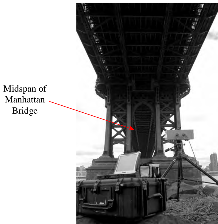
Figure 9. IBIS-S installation during the Manhattan bridge demonstration test from the Brooklyn side
