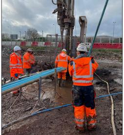
Standard sized boreholes (120mm diameter) were drilled relevant to the 70mm inclinometer casing and magnets, the annulus grouted in place - https://www.geosense. co.uk/grout-calculator - datalogged via a digitial node into a position of safety.
