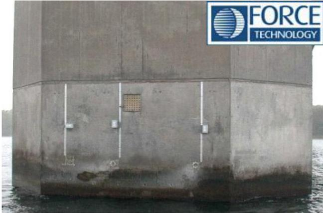
Figure 1. CorroRisk probes mounted on bridge pillar
