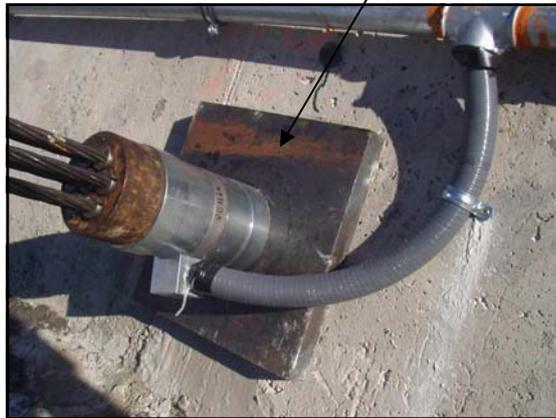
4. Place the base load distribution plate over the anchor strands or bolt followed by the cell and then the top load distribution plate.
