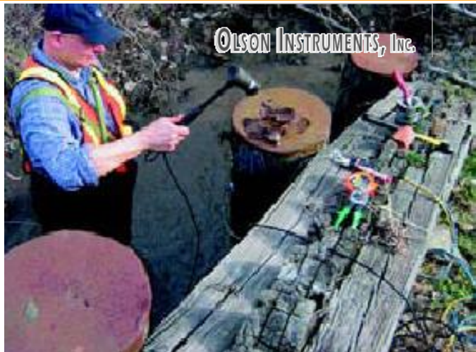
Figure 1: Testing using the Ultraseismic method
