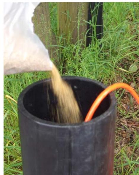
12. Pull the temporary casing back to the elevation of the top of the filter and add more clean filter sand on top of the piezometer. Continually check the level of the sand using the weighted tape.
